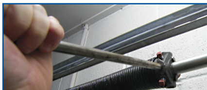
Attach pre-set torsion assembly, spacer bar and wind spring.
