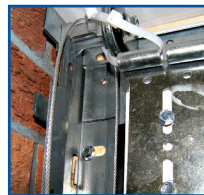
Lift into opening, level, fit top corner fasteners and lock top section.
